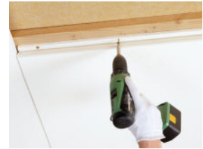
Master F is installed by screw fixing
