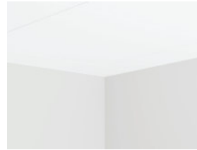
Sealed junction with wall
