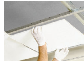
The individual tiles are easily demountable
