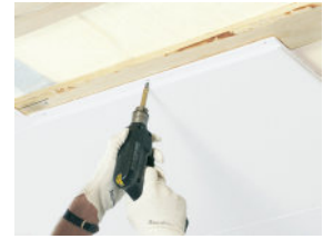
Focus F is installed by screw fixing
