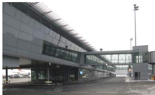
International Airport, Riga_Latvia product installed: Open Cell BASE 15 H 38 > 150X150 MM surface: 13.000 sqm.
